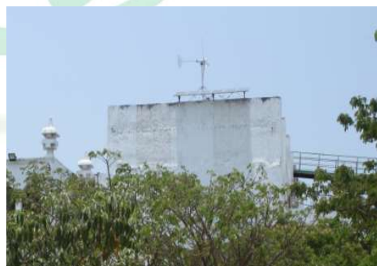
Figure 49: Solar-Wind Hybrid system
