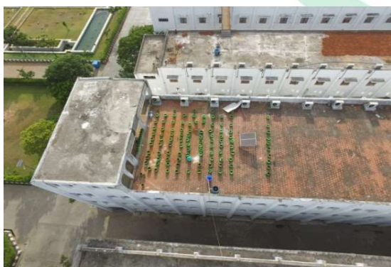
Figure 48: Roof top solar panel
